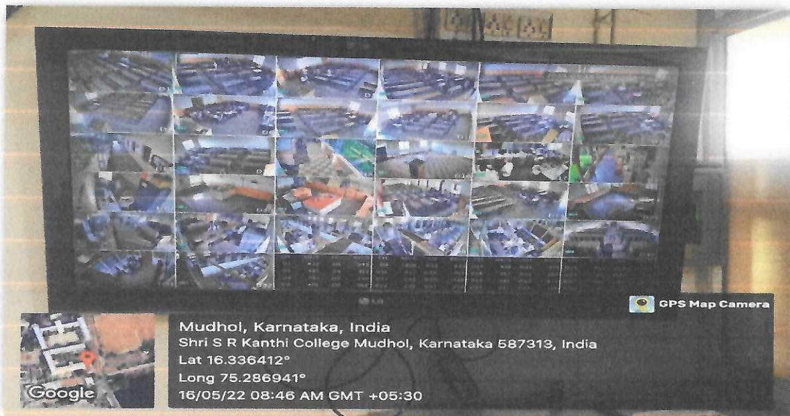
CCTV'S VIEW AT CHAMBER
