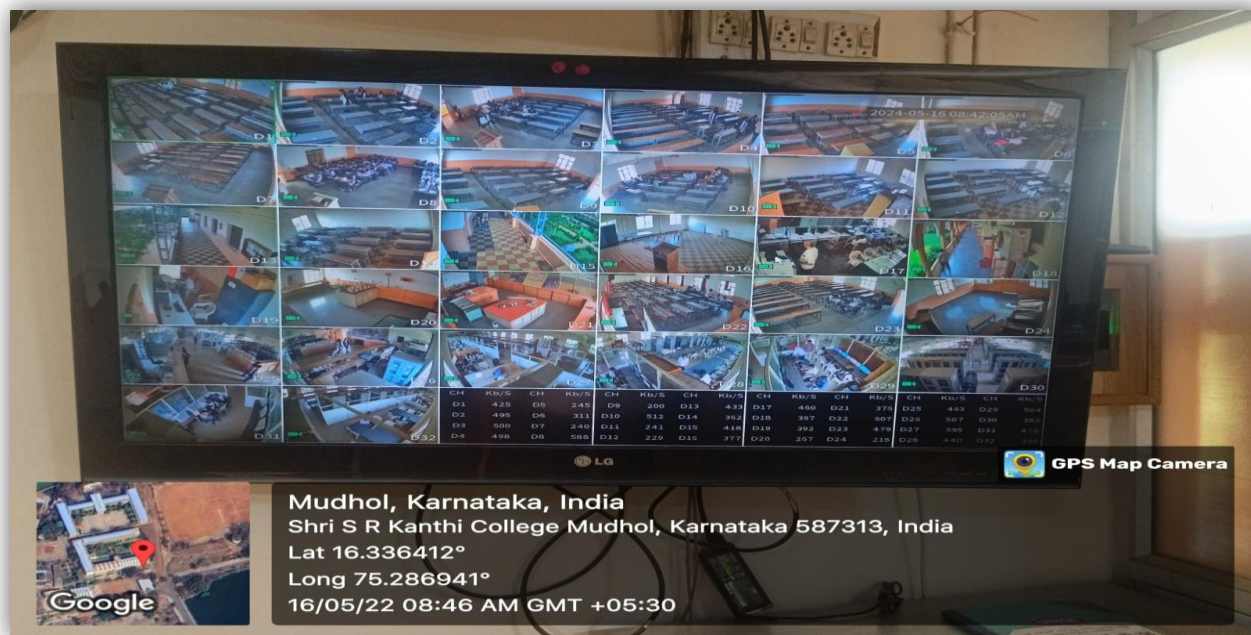
CCTV'S VIEW AT CHAMBER
